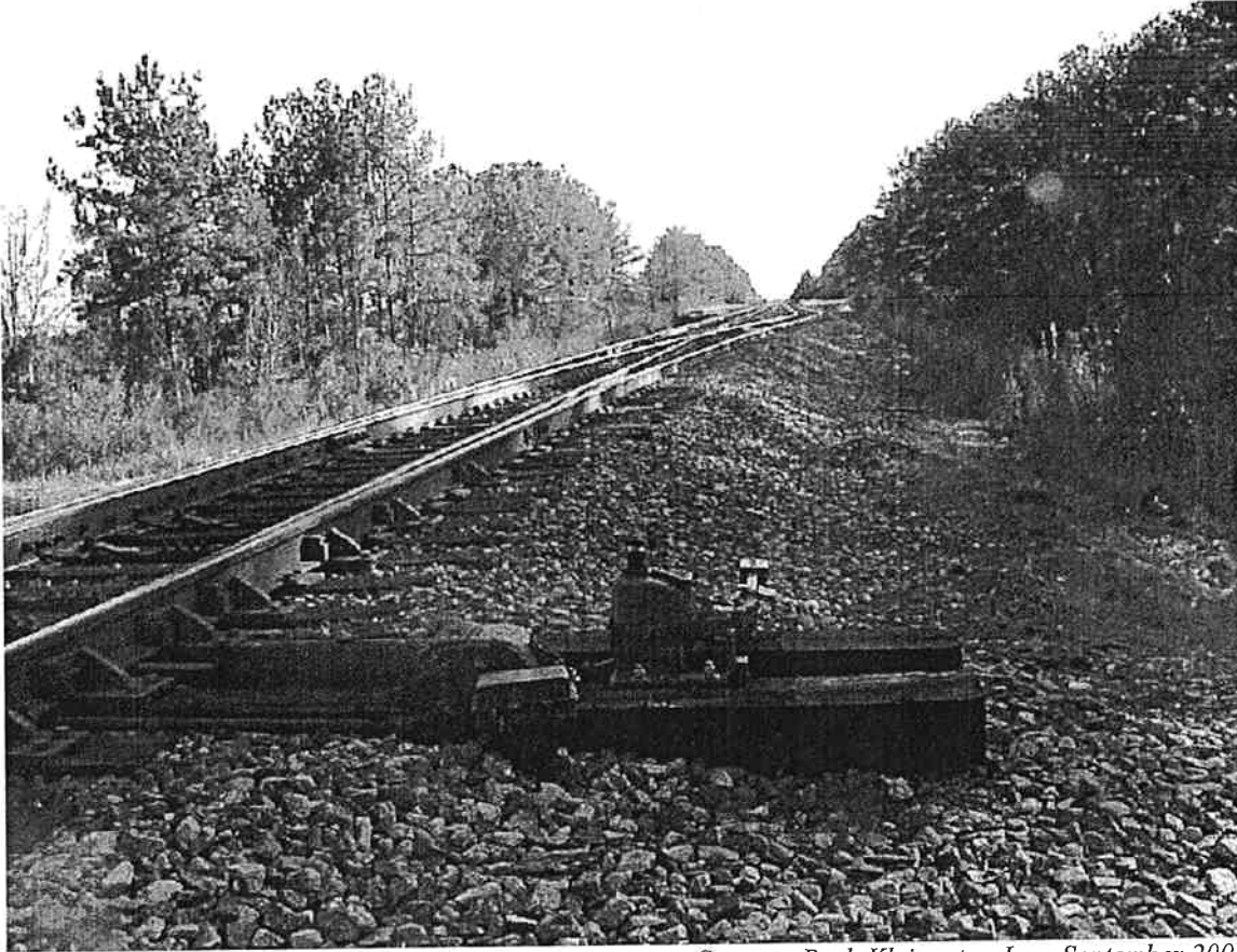
Figure 4-9: Hand thrown No. 10 Turnout at south end of Barnett Siding
