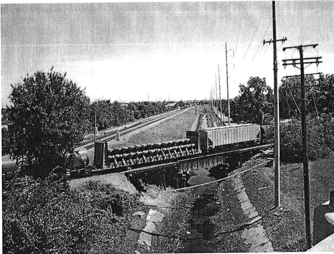
Figure 4-18: SB freight on CS Track 2 over drainage canal. NB Norfolk Southern train in distance.
