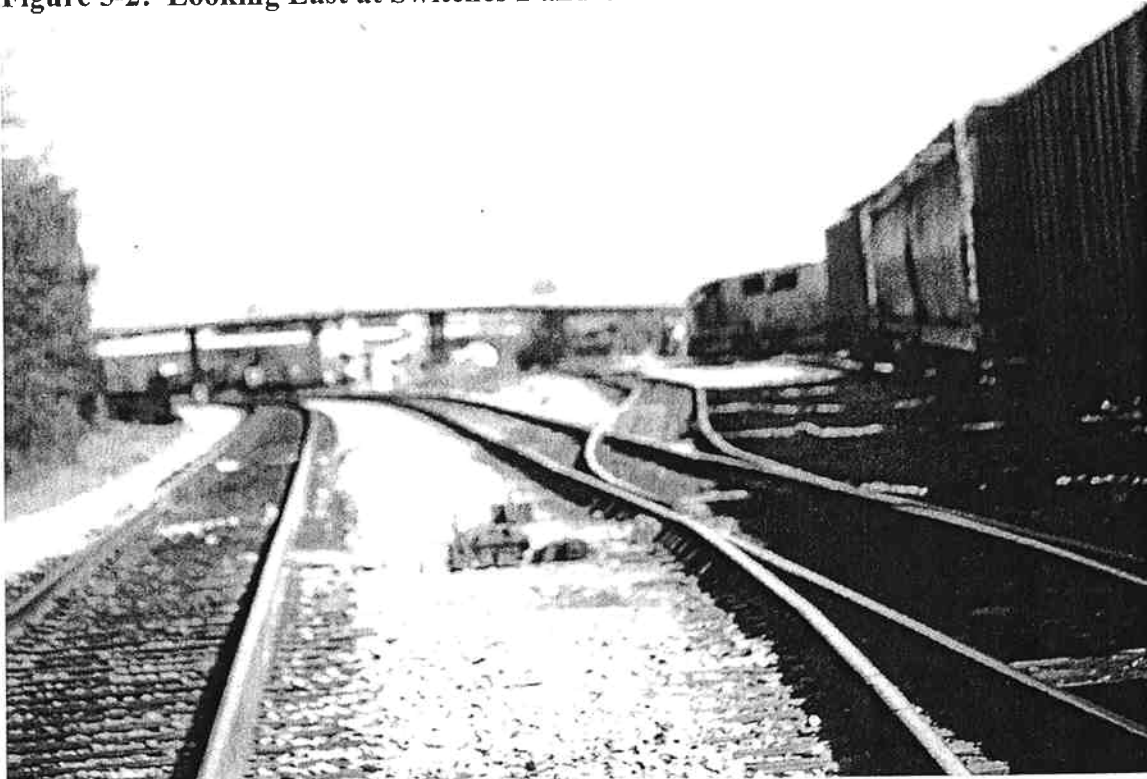
Figure 5-2: Looking East at Switches 2 and 4
